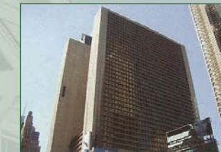
THE MARRIOTT MARQUIS PIPE CHASE
