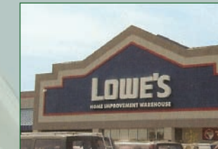
CEMENT BLOCK CONSTRUCTION
