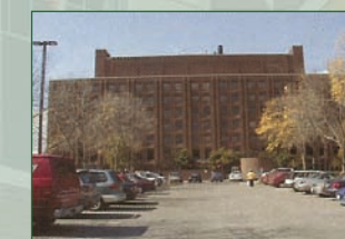
MEDICAL CENTER LABORATORY INSULATION
